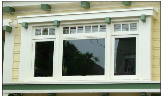
**Vinyl:** Vinyl windows are made primarily of polyvinyl chloride (PVC), a product that offers many advantages. This type of window typically looks heavier than a wood or metal window because vinyl is not strong enough to be made into ultra-thin parts, and the texture is unmistakably plastic. Except for washing the glass, maintenance is a breeze and is typically free from recurring service – painting for example.
